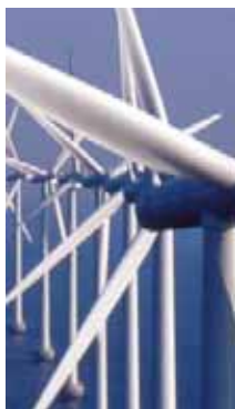
Middlegrunden Offshore Wind Farm Photograph by Mads Eskesen
